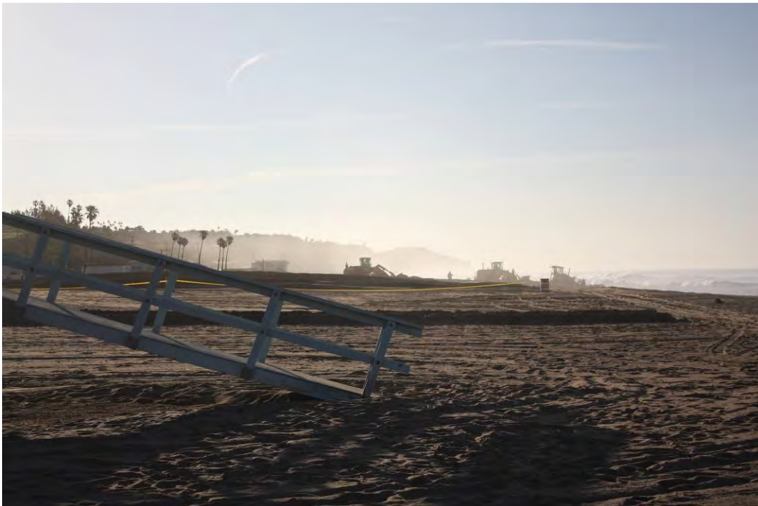
Photograph 18. Sand replenishment project south of LT 9.
